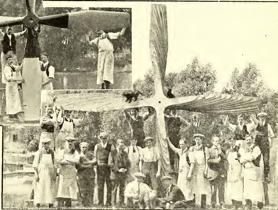
MUNITIONS OF WAR.— A Lang Propeller for a British Aircraft. It is here shown in its finished and unfinished state, together with some of the men who made it. It is the biggest single-piece four-blader on record.
